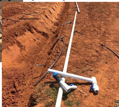
(Below) Underground Micro-Irrigation during installation
