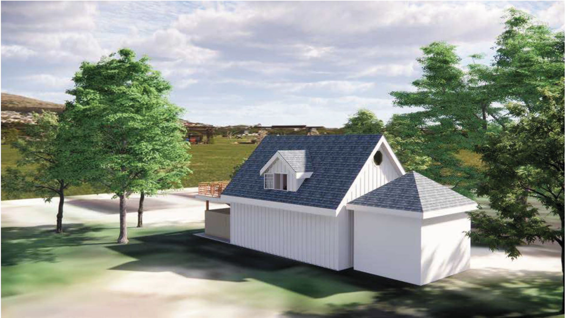
Back Facade - Aerial View
