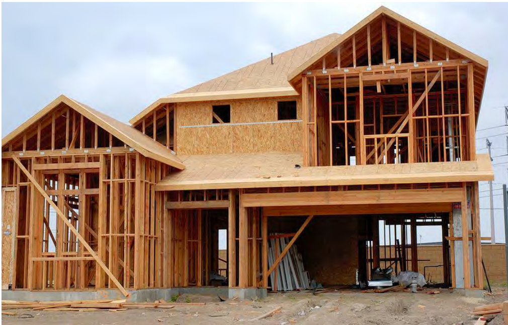
UC- Under Construction
