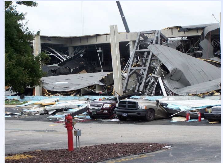
ConAgra National Gas Explosion and Ammonia Release, June 2009 Garner, NC
