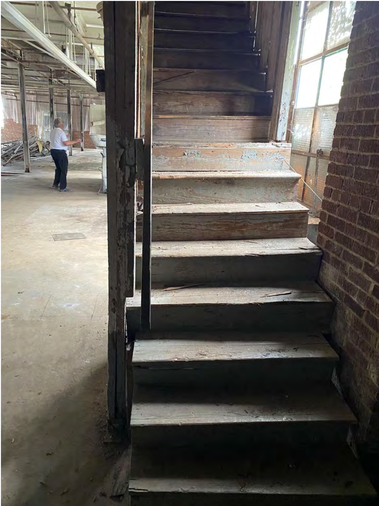
First level, stair
