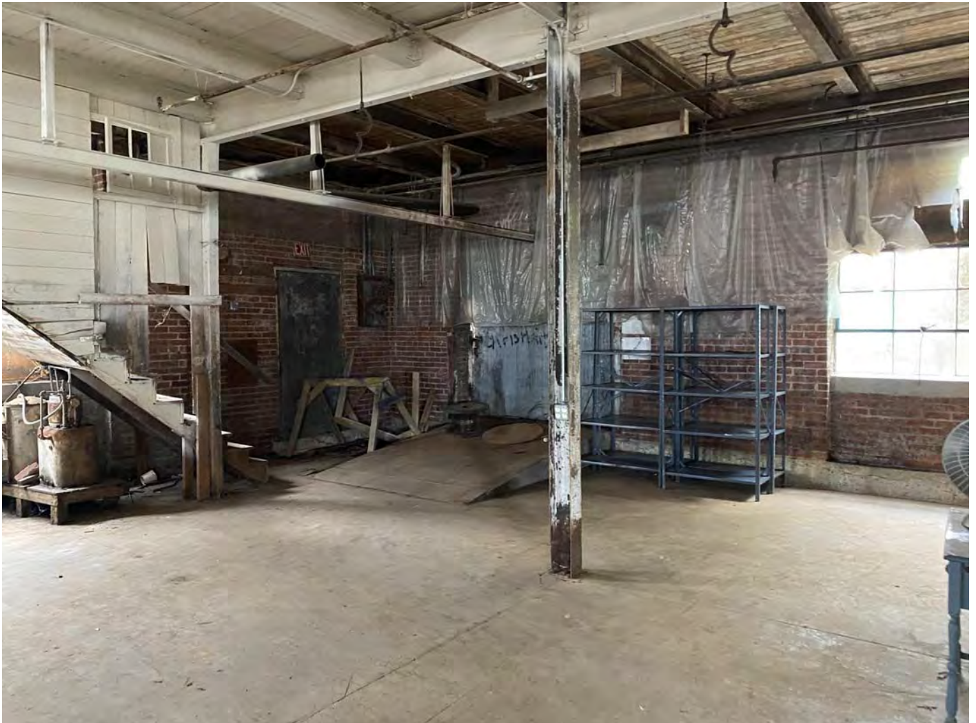
First level, rear elevation door
