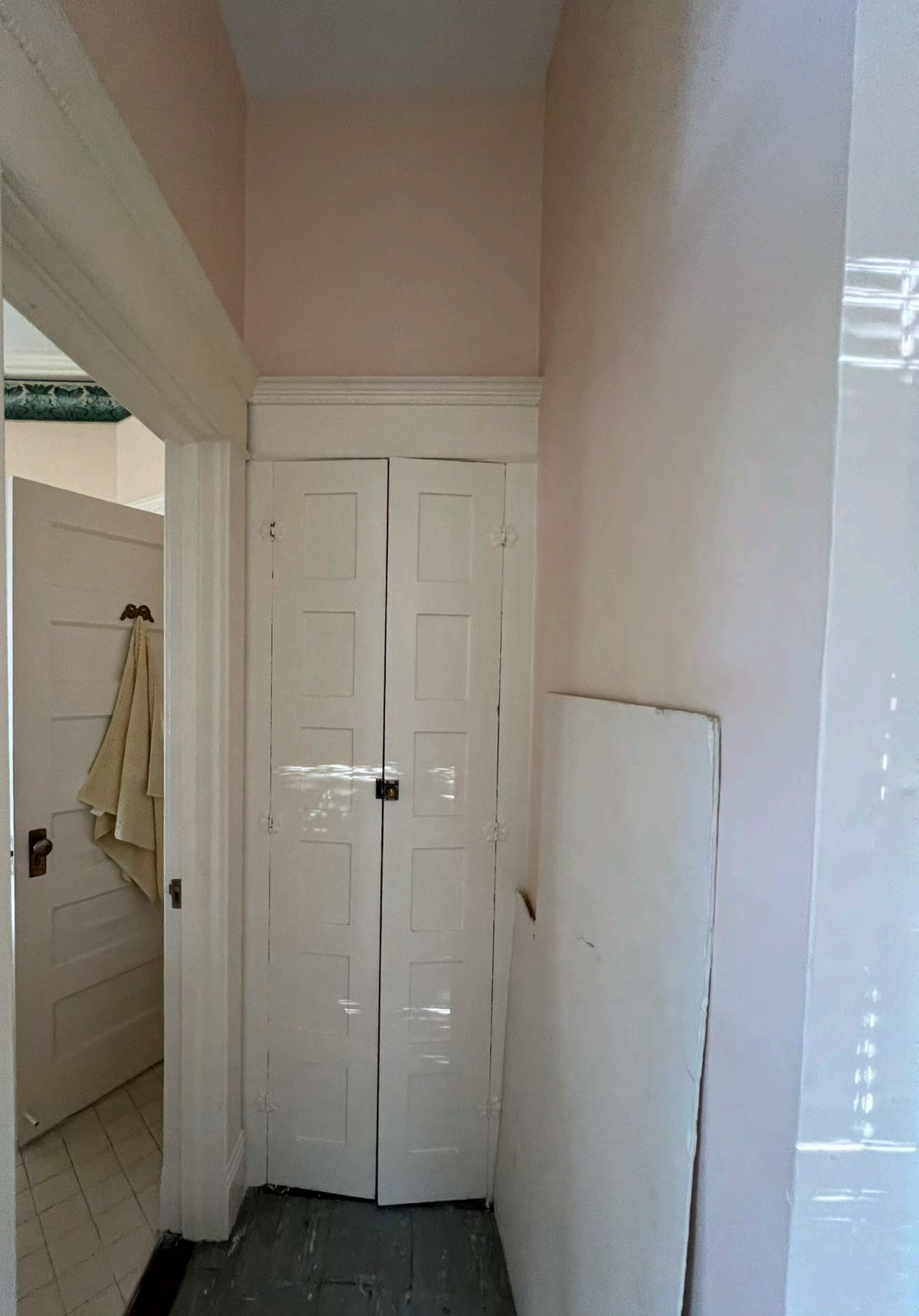
Door and closet to be removed
