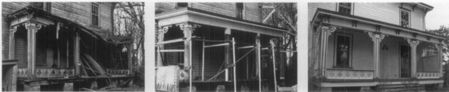
Figure 5. Even historic porches that appear to be in total disrepair may be repairable. While the roof needed replacement, much of this porch was repaired, including such features as the decorative columns, ornamental brackets, and balustrade. Photos: John Leeke.
