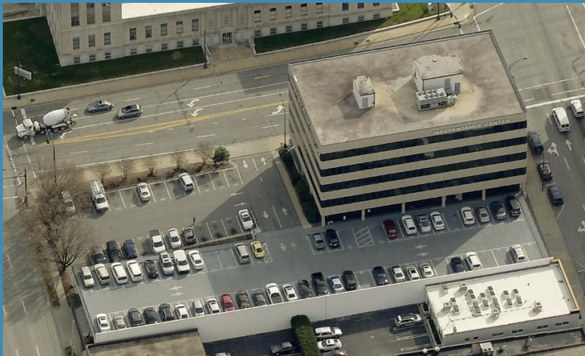
View From the West
