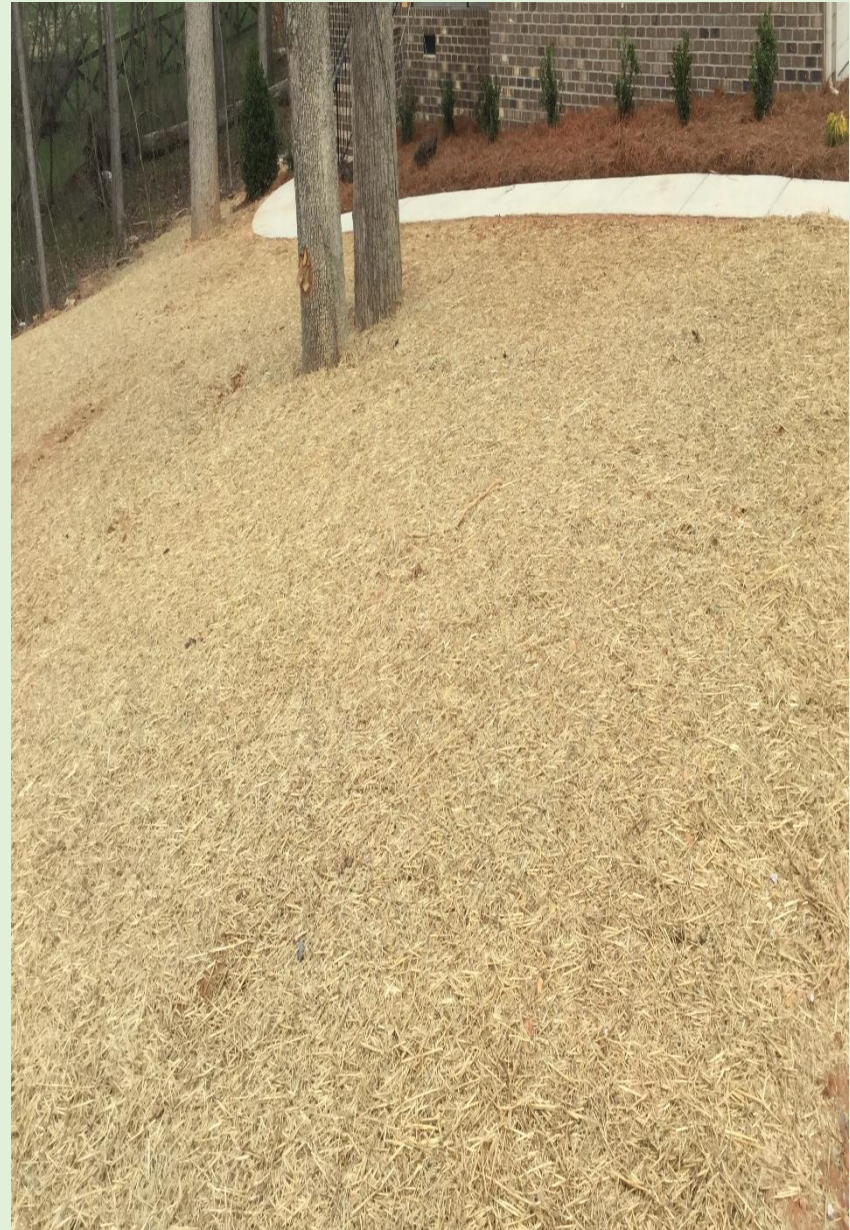
Permanent seeding stabilizes disturbed areas with vegetation for periods longer than 12 months. Temporary seeding stabilizes disturbed areas before final grading, or in a season not suitable for permanent seeding.
